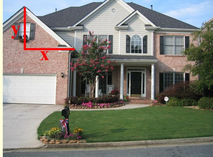
Builders need to know the pitch of a roof to determine which type of shingle will be appropriate for the roof.
